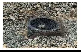
around the pipe stub with geotextile and rock.
