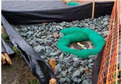
extremely important (it can be square or triangular), it is a good idea to include geotextile fabric inside the silt fenced area and cover it with some rock. (This particular photo also includes a compost sock or Type 7.) However, please remember that silt fence is not very permeable and you could get some flooding outside it. TIP: to alleviate this, make the fence perimeter longer which allows more linear feet of fence to accommodate a higher pass-through flow rate.
