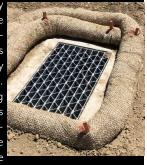
the fiber roll perimeter than outside the perimeter where all the "untreated" water is. This is caused by the turbulent water jetting under or cascading over the fiber roll. It should be noted that CASQA does not include fiber rolls in their BMP fact sheets as a DI protection option. Check out this video for more information on this phenomenon and a better DI protection option.
