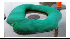
socks will typically reduce turbidity numbers, there are limitations to where compost socks can be used. They are not ideal for areas of high traffic-although they can handle being run over by a pickup truck or car, heavy equipment will usually destroy them in a couple of passes. They are best suited for paved or smooth compacted soil surfaces—unless you stack them up, loose non-compacted soil can overwhelm them.
